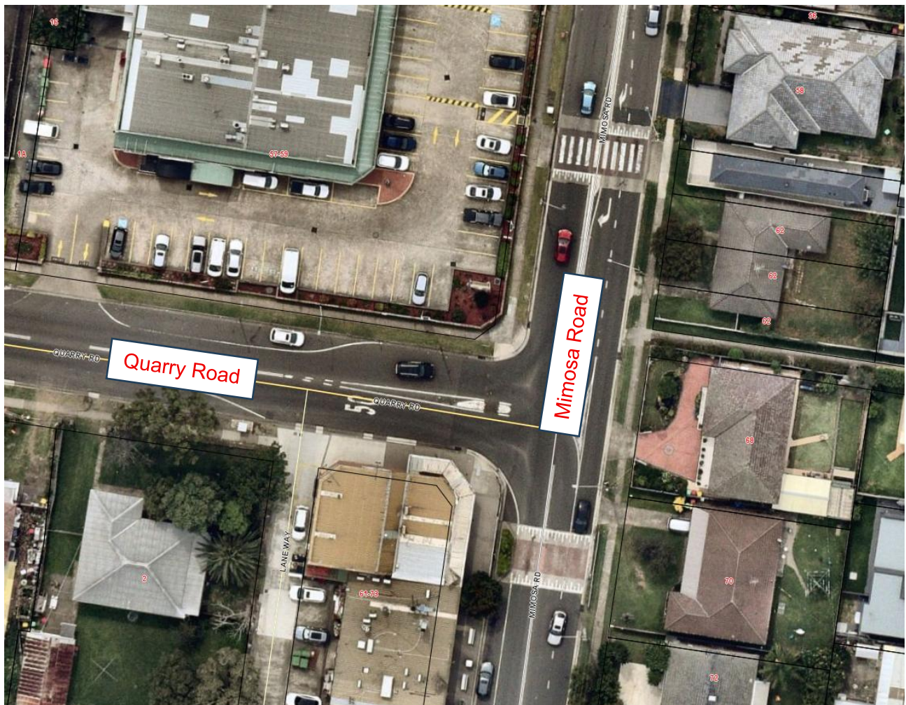
Figure 1: Aerial image of the T-intersection of Mimosa Road and Quarry Road Bossley Park
