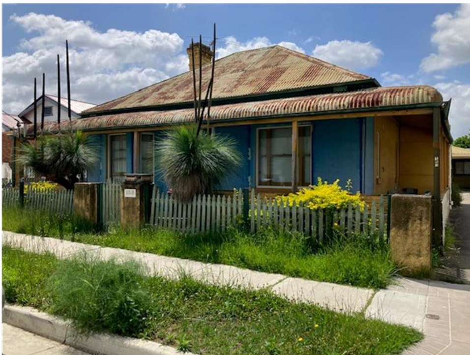
Figure 12 -Front (west) elevation of of 158 Broomfield Street.
