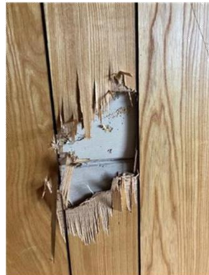
Figure 42: Wall cladding underlain.
