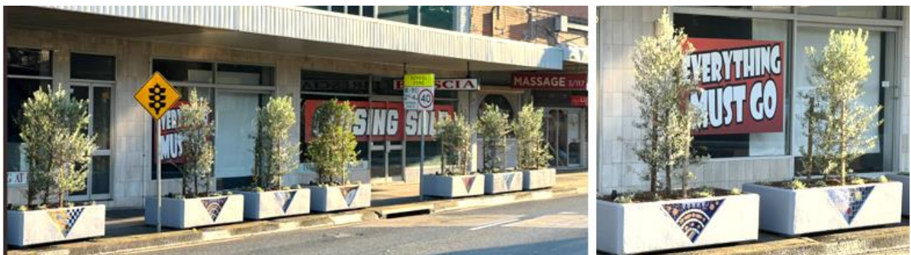
Planter box upgrade, Cabramatta Road East Cabramatta.
