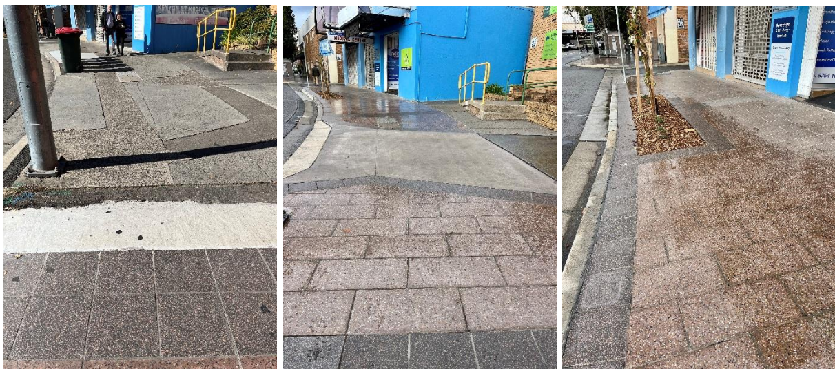
Before and after shots of Kenyon Street Pavement Project.
