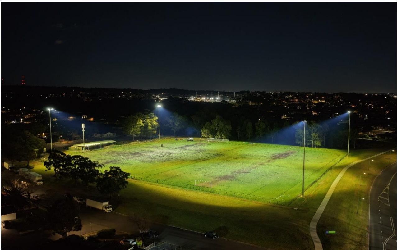
Figure 2 Stage 1& 2: Floodlights installed and operational.
