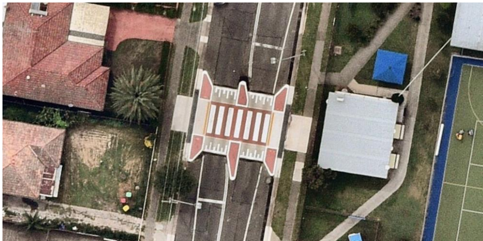
Newly replaced pedestrian crossing in Cumberland Street, Cabramatta
