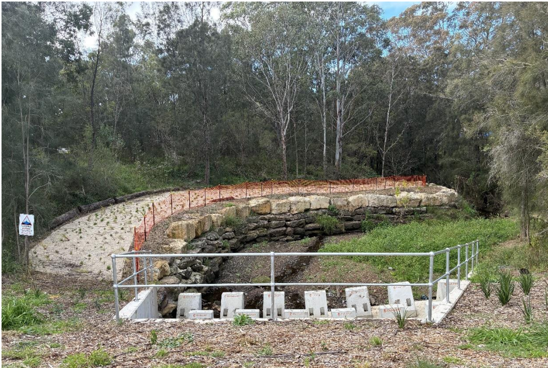
Figure 4 Bank stabilisation and planting downstream of Powhatan Reserve Detention Basin
