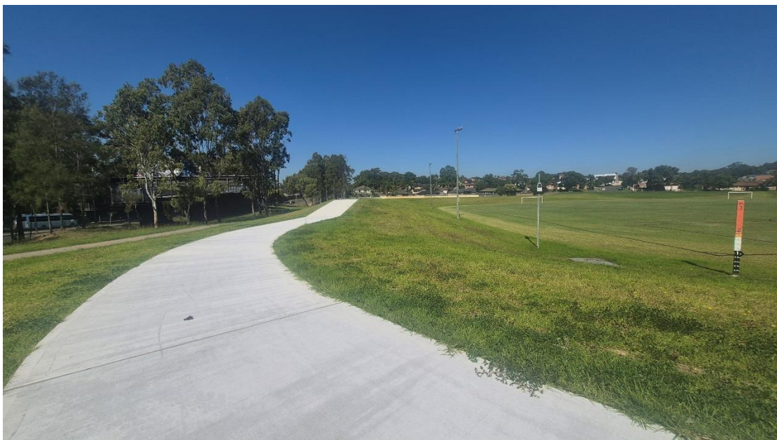
Figure 6 Concrete spillway at Stockdale Reserve Detention Basin
