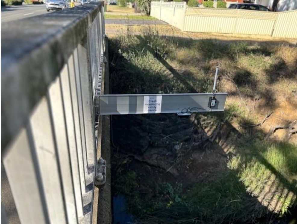
Figure 1 Water level gauge
