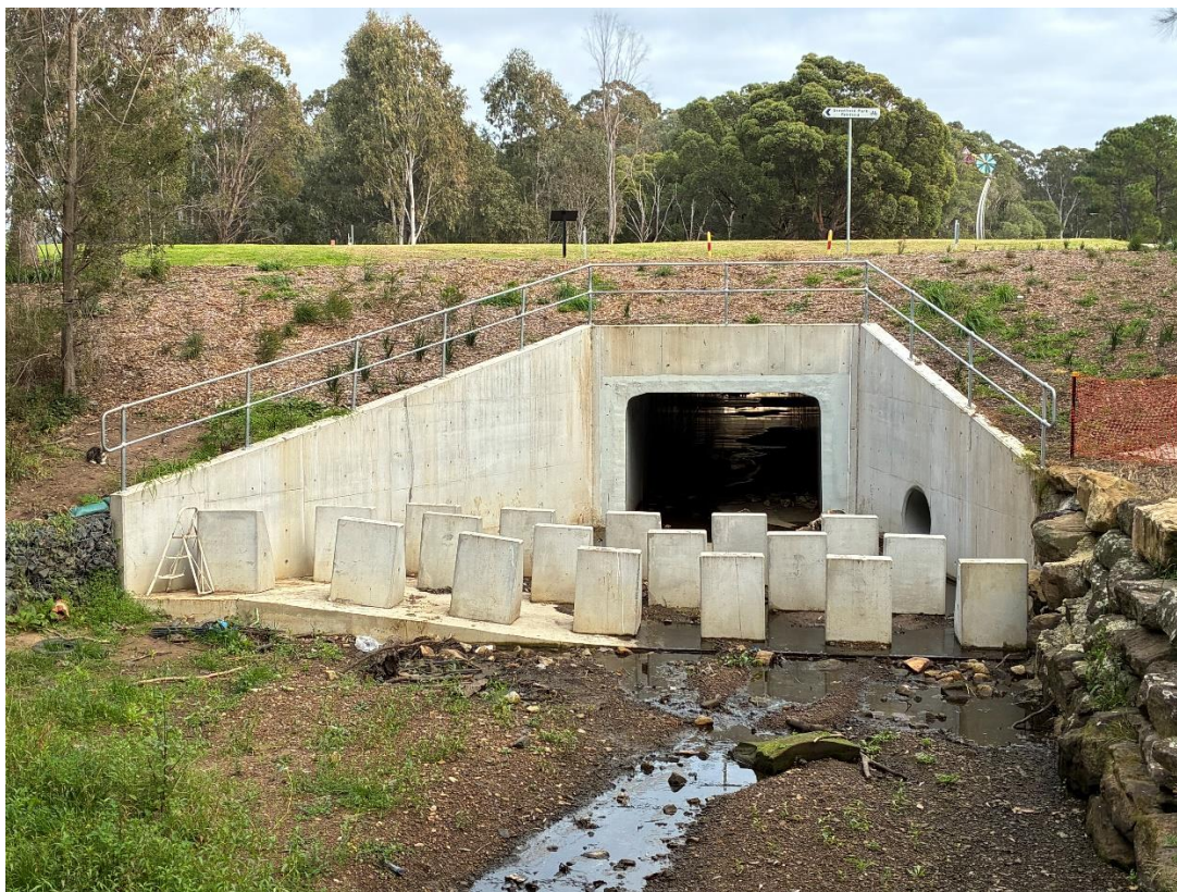
Figure 3 Energy dissipation baffles downstream of Powhatan Reserve Detention Basin
