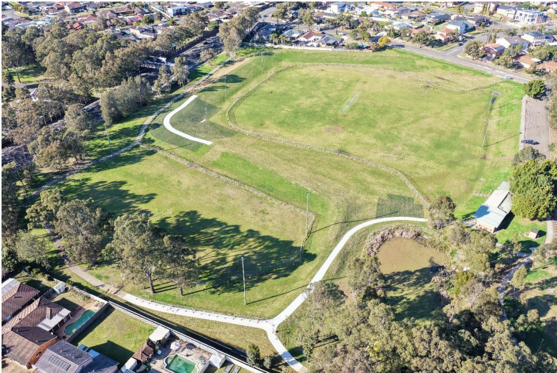
Figure 5 Aerial view of Stockdale Reserve Detention Basin
