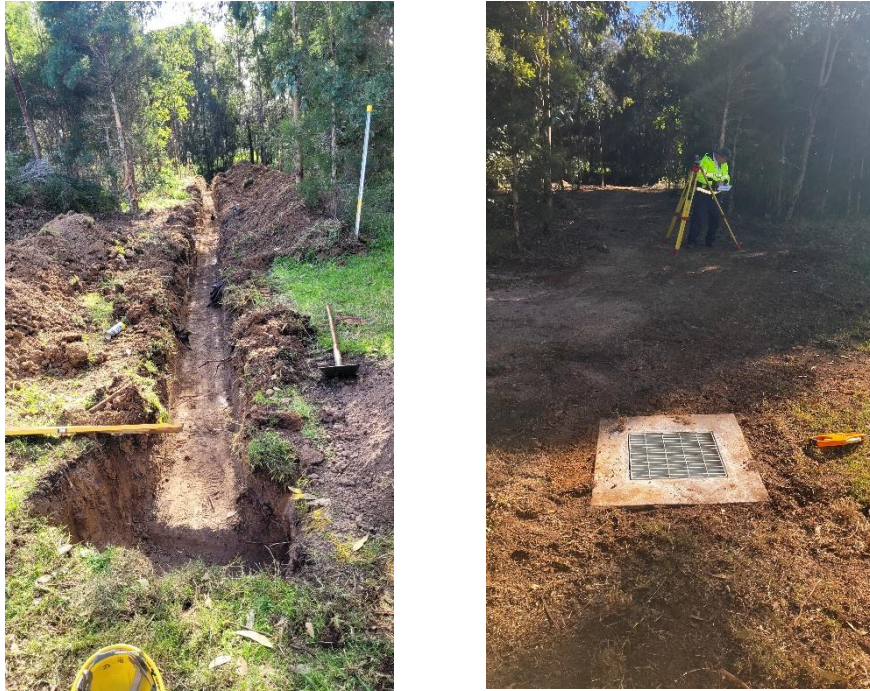
Figure 7 Barook Place Mount Pritchard Drainage Improvements
