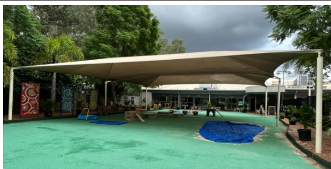
Figure 6 – Wetherill Park ELC shade sails after replacement.
