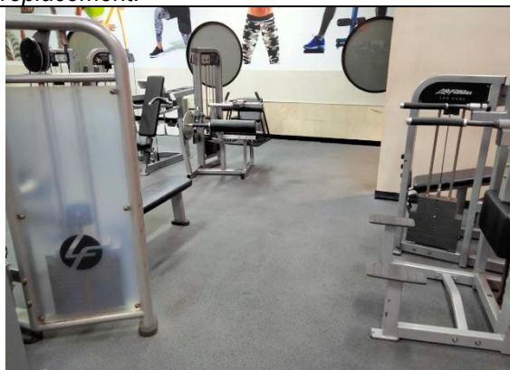
Figure 7 – PLC Gym flooring before.
