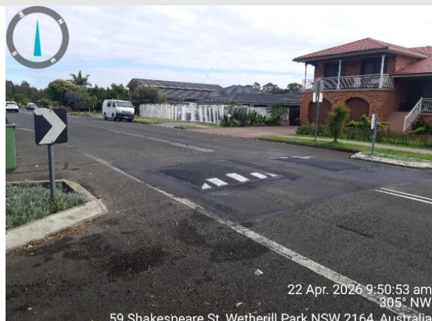
MPTFR2618 - Shakespeare Street, Rubber Cushions and Islands between Gower Close and Otway Close
