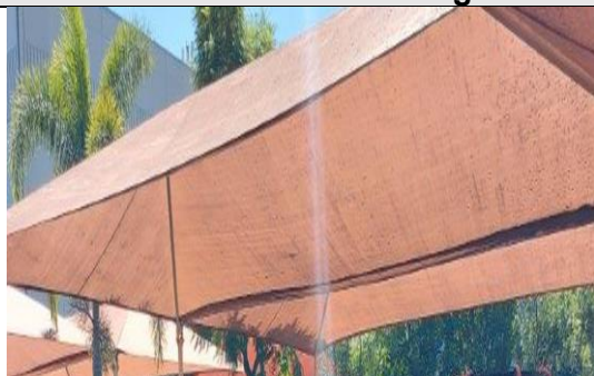
Figure 5 – Wetherill Park ELC shade sails before replacement.
