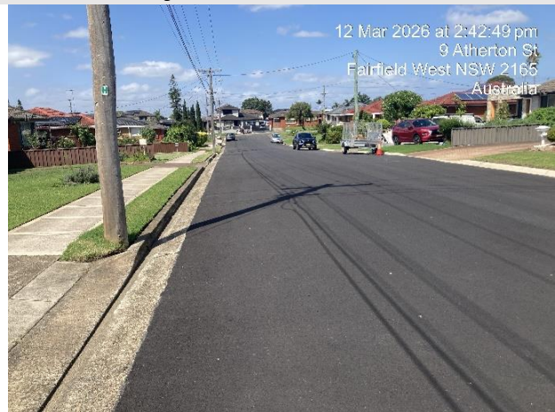
Resurfacing – MPRR2638 – Atherton Street - from Cambewarra Road to Hamersley Street
