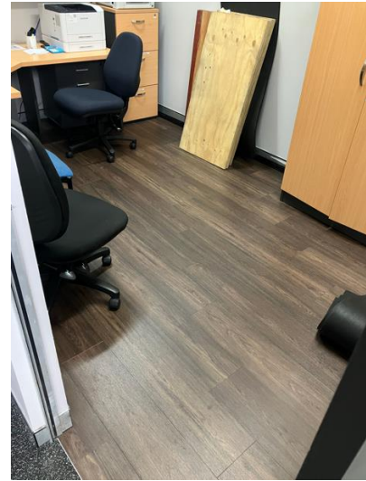
Gym office vinyl install.
