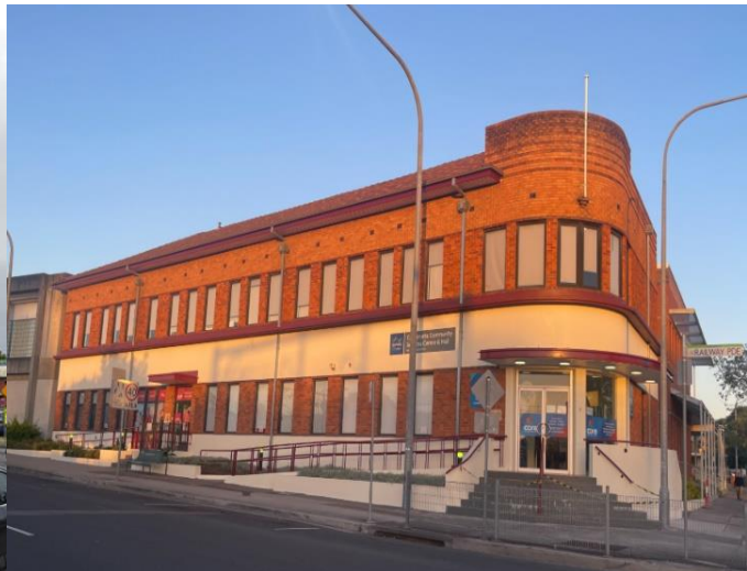
Figure 2 – After façade works completed.
