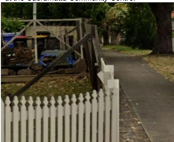
Figure 3 – 76 Chifley Street Smithfield before fencing replacement.
