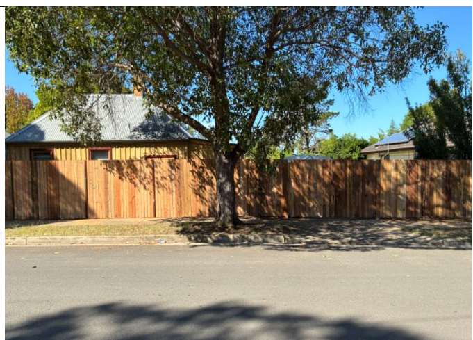
Figure 4 – After fencing replacement.
