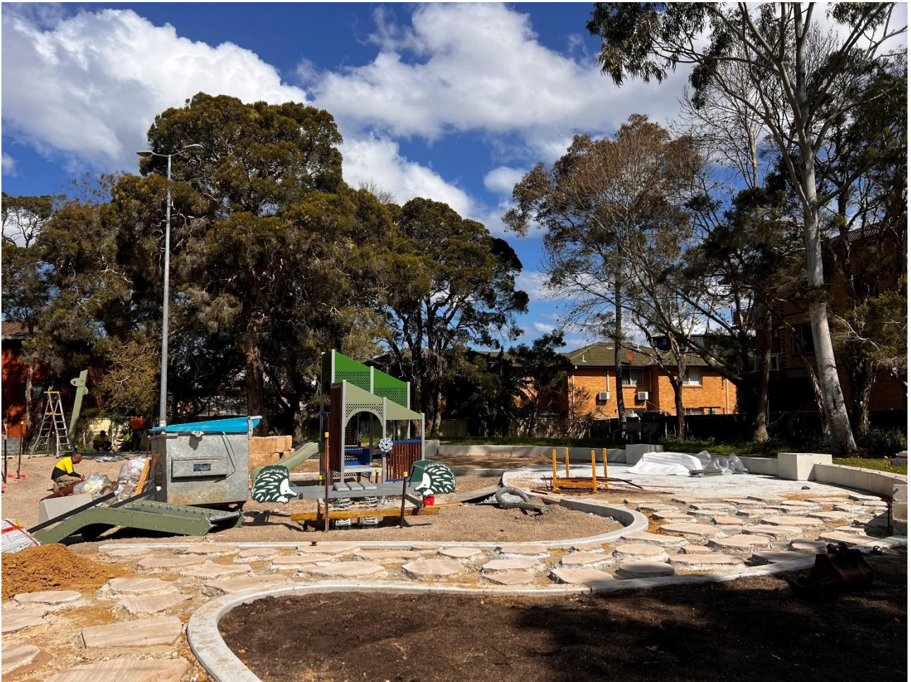
Figure Nelson 2: Nelson Park Construction Site
