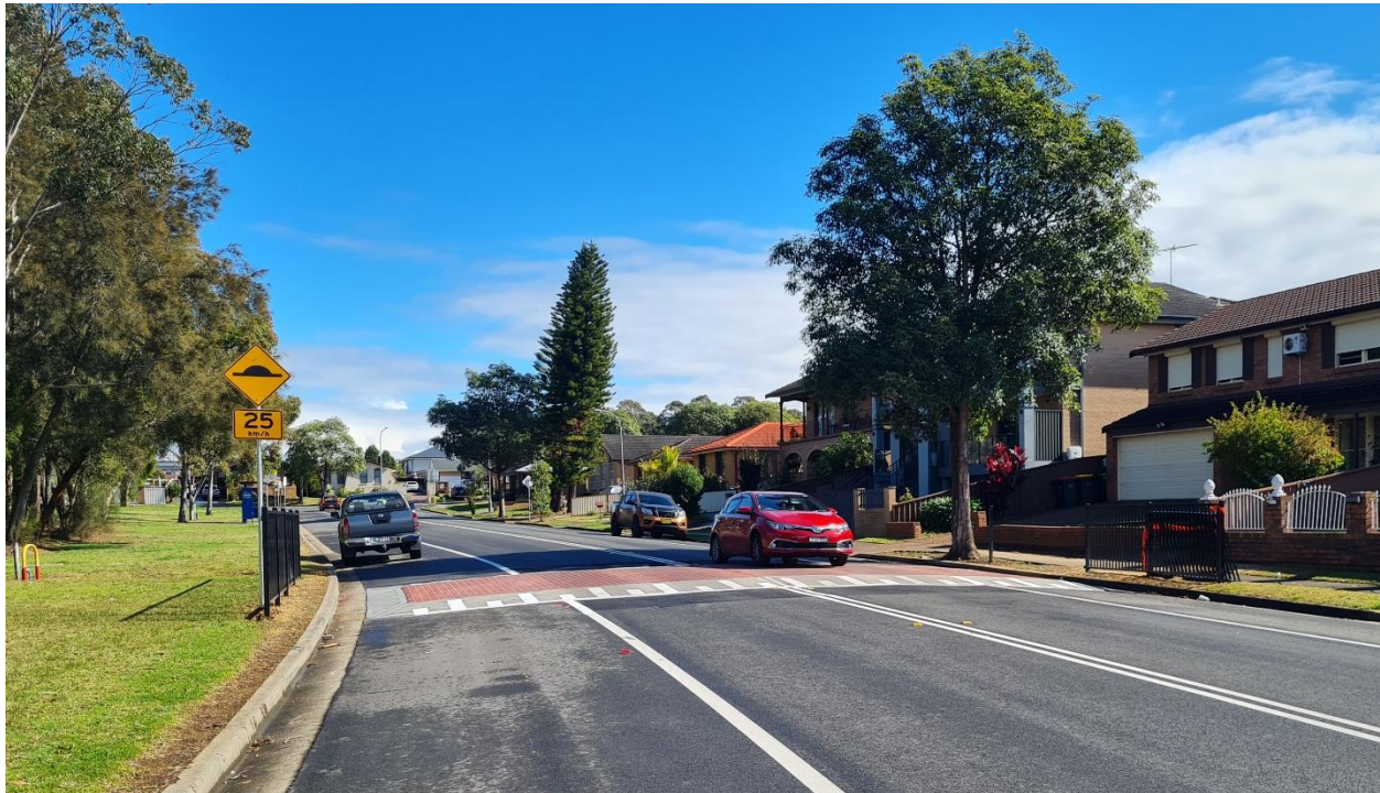
New raised threshold along Shakespeare Street Wetherill Park.
